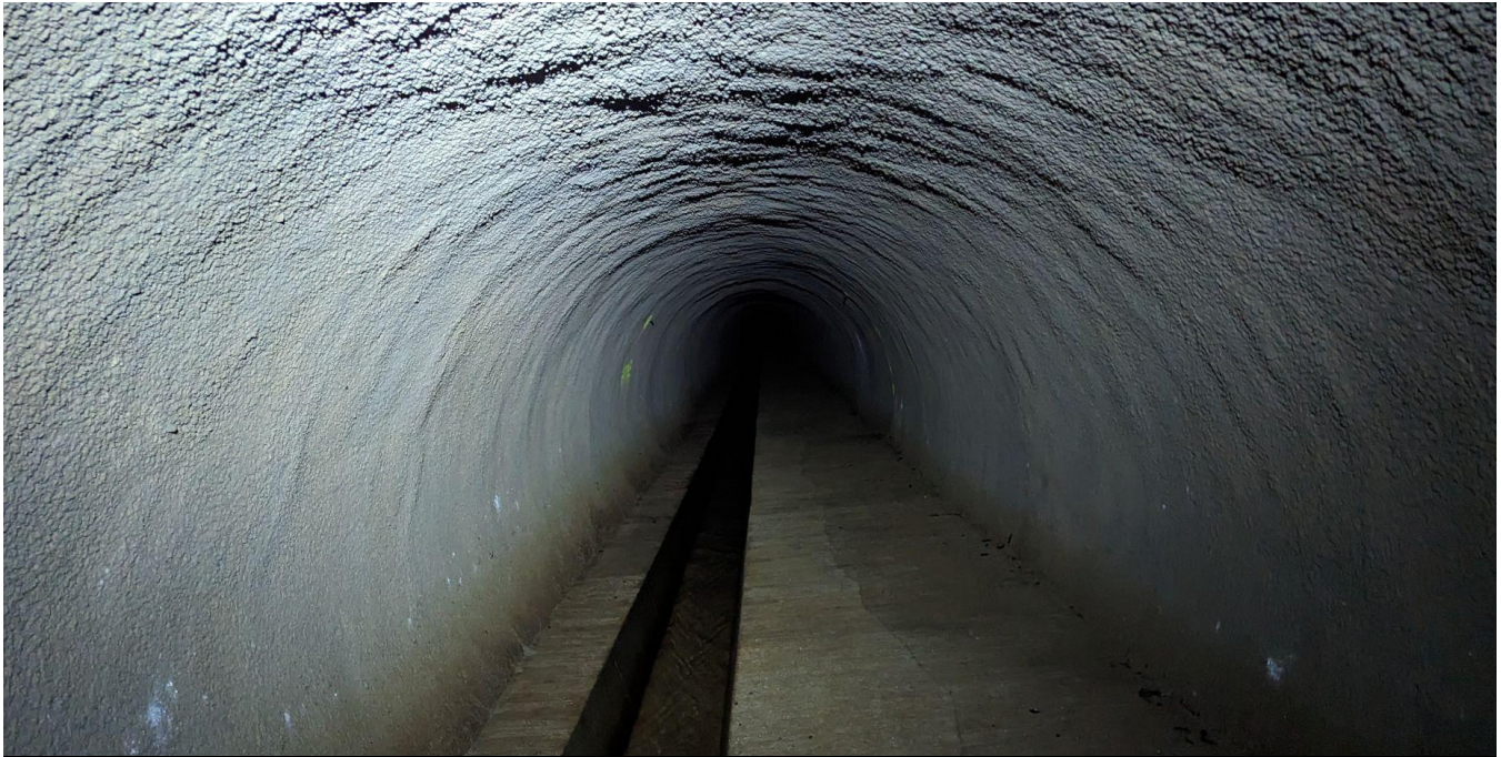
The variety of geometric features in this corridor meant that drift was reduced This tunnel has little to no clear geometric features to help reduce drift in a LiDAR scan
