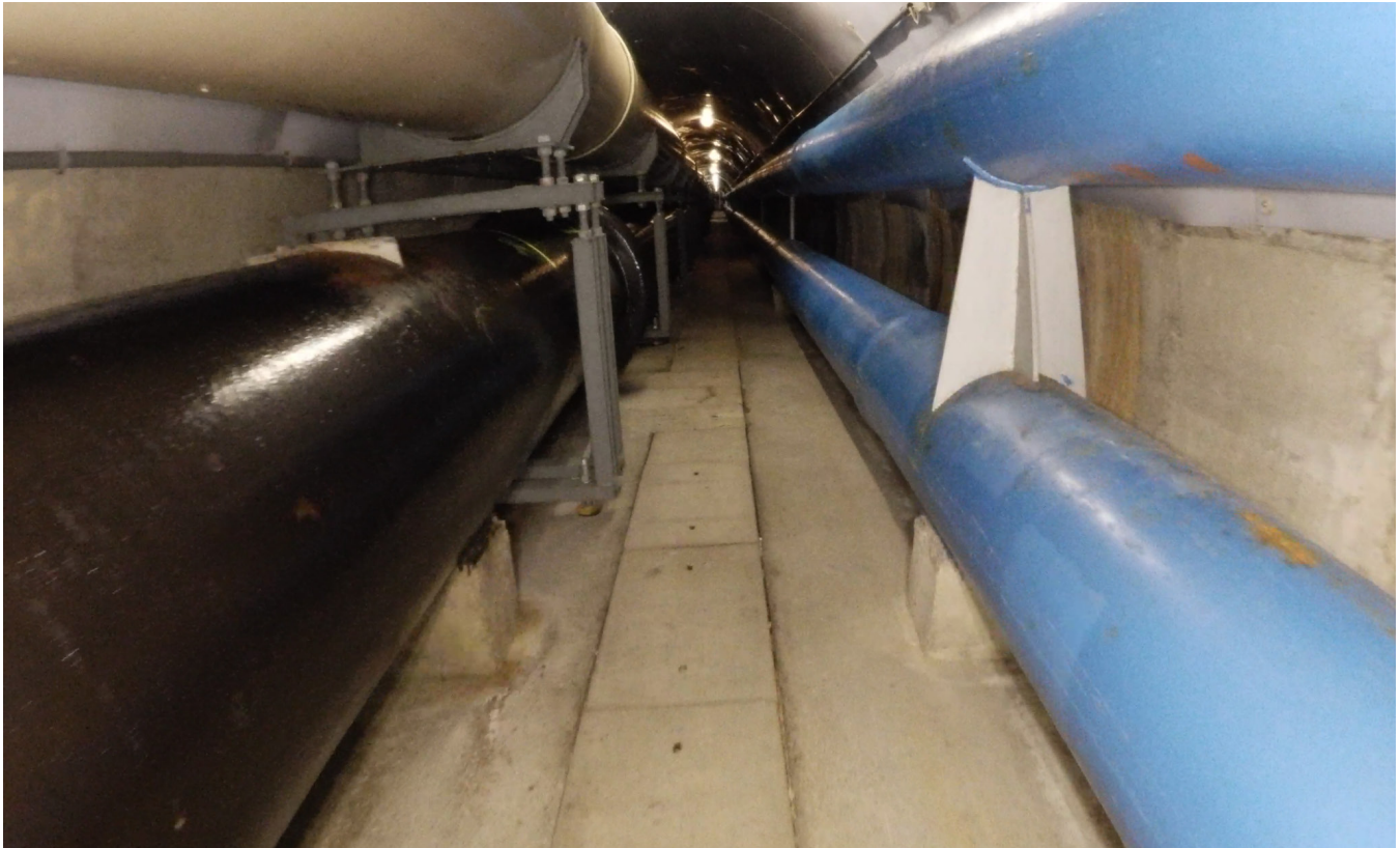
The variety of geometric features in this corridor meant that drift was reduced
